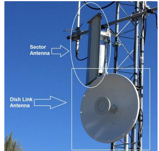
Signal Peak node antennas.
