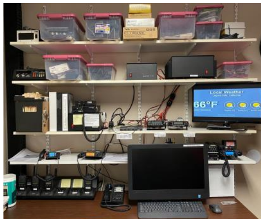
Laguna Woods RACES radio area at City Hall.
